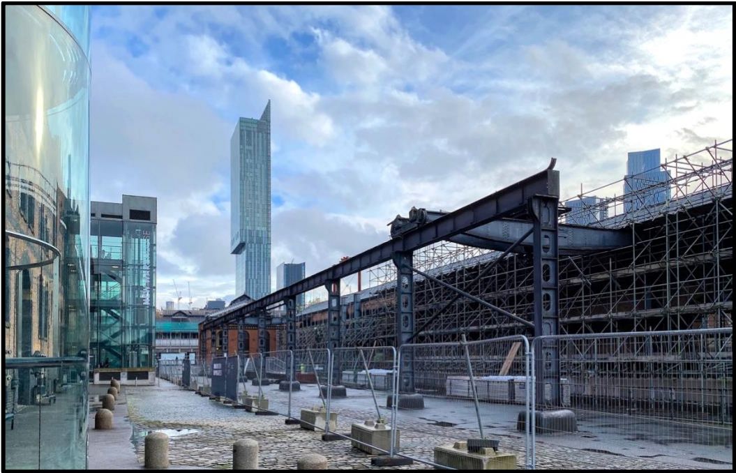
MOSI Power Hall under renovation
