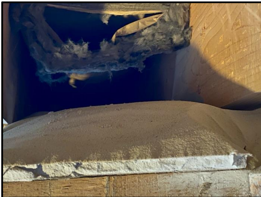
The sand over the top surface of the 3 layers of plasterboard.
